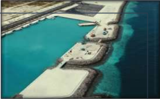
VIA SW Harbour
